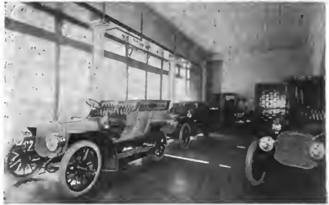
MAIN SALESROOM, FIRST FLOOR, NEW LOZIER STORE.
